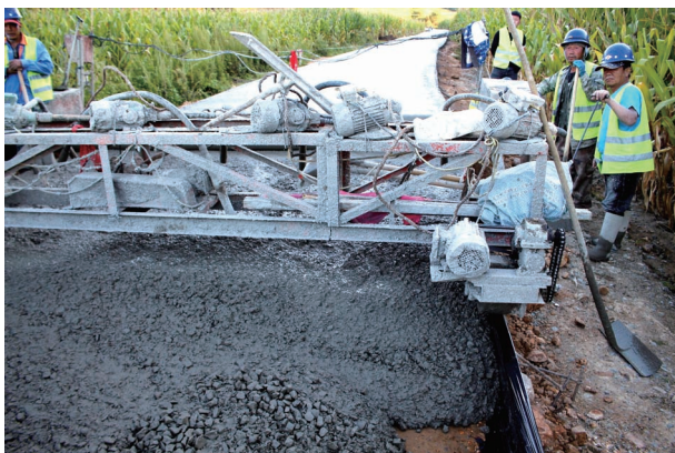
“四好农村路”施工现场
